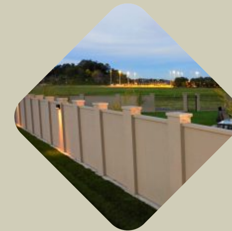
Secured Compound Wall
