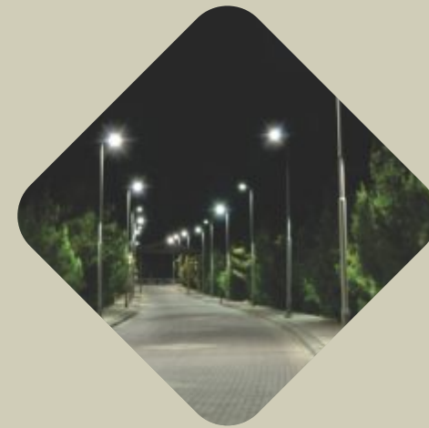
Street Lights & Rainwater Trench
