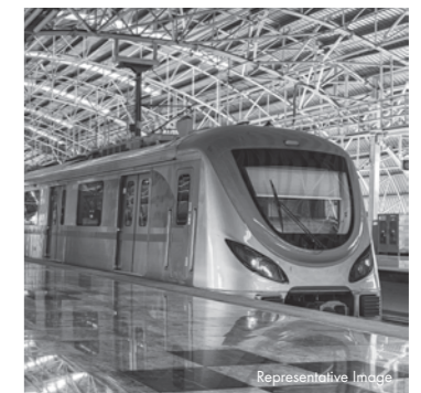
Erected Bangalore Metro Car Shed.
