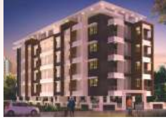
RAMAKRISHNA RESIDENCY Paduva Mangalore
