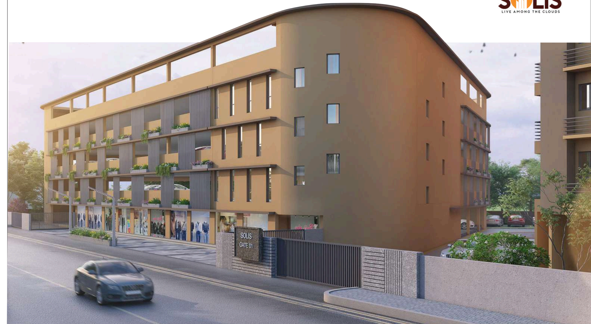
VIEW OF PARKING BLOCK
