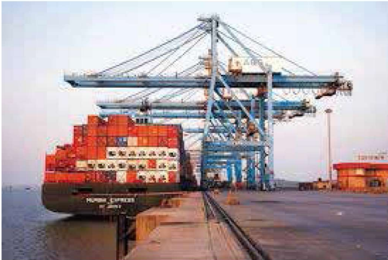
New shipping terminal near Dahanu
