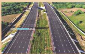
6-Lane Bangalore Highway (NH-44)
