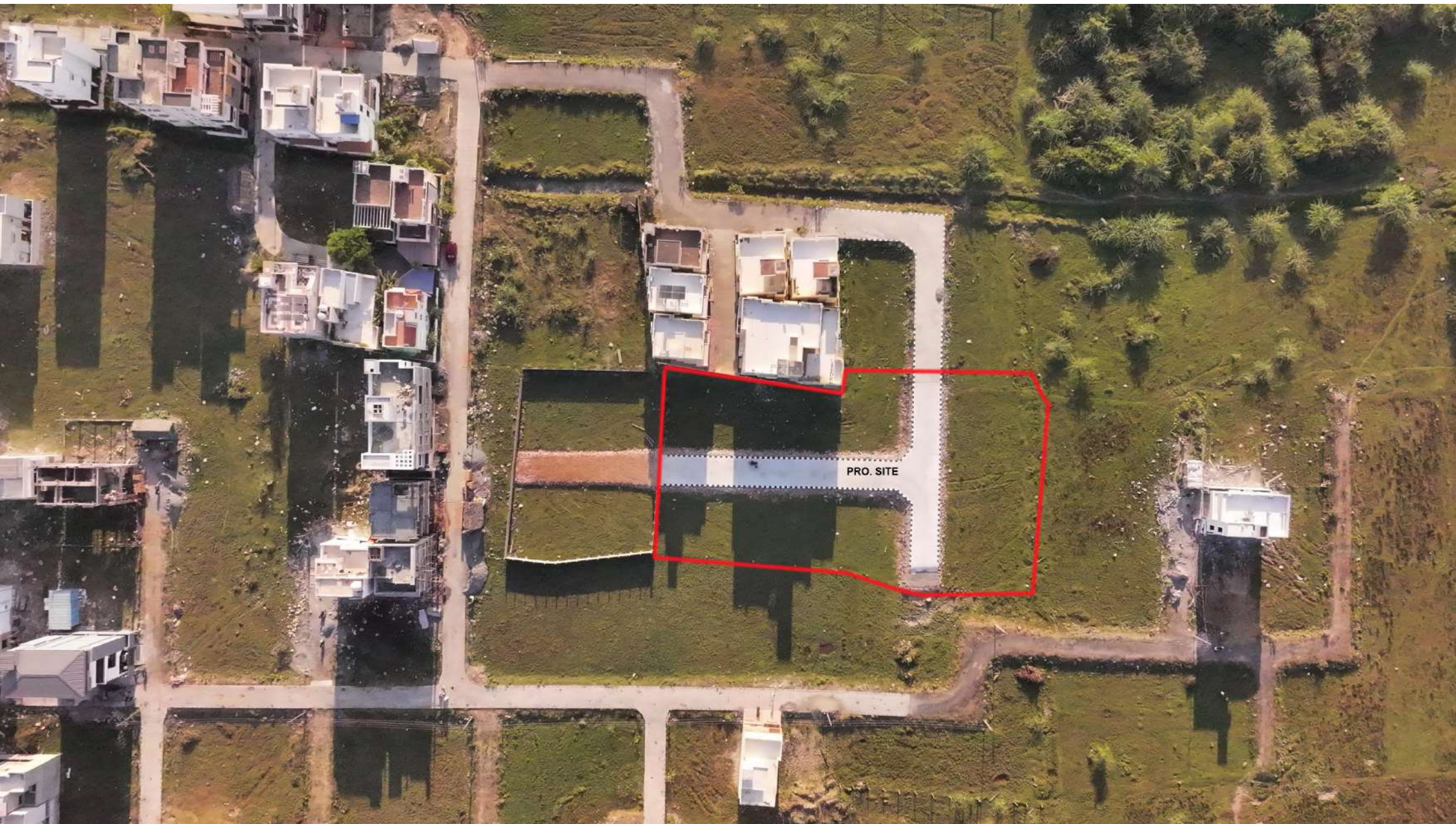
DRONE TOP VIEW
