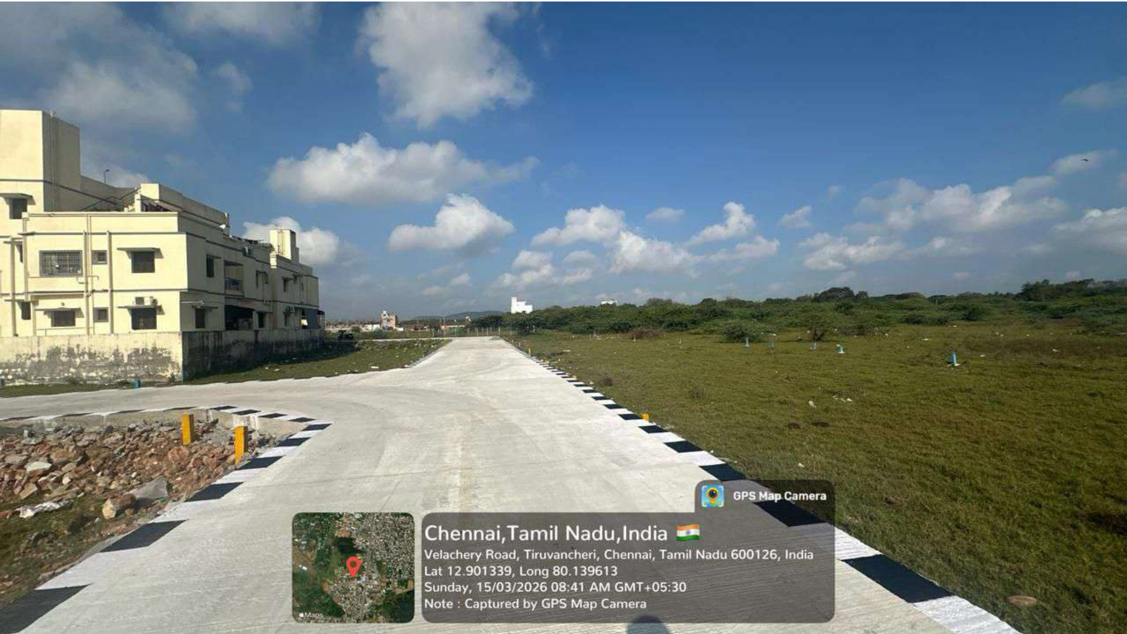
WEST SIDE VIEW
