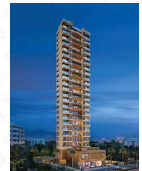
DREAM AVENUE Khadakpada, Kalyan (W) 22-Storeyed Residential Landmark
