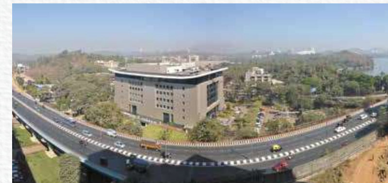
30 Minutes To The International Airport Via JVLR & Andheri Kurla Road.
