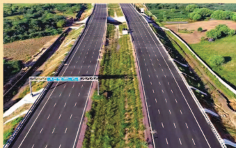
6-Lane Bangalore Highway (NH-44)
