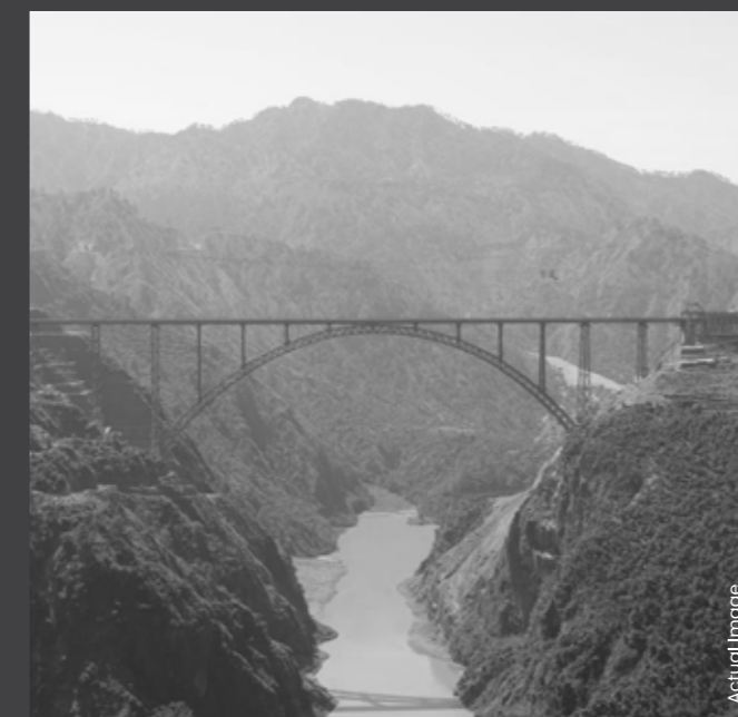
CHENAB BRIDGE, J&K
